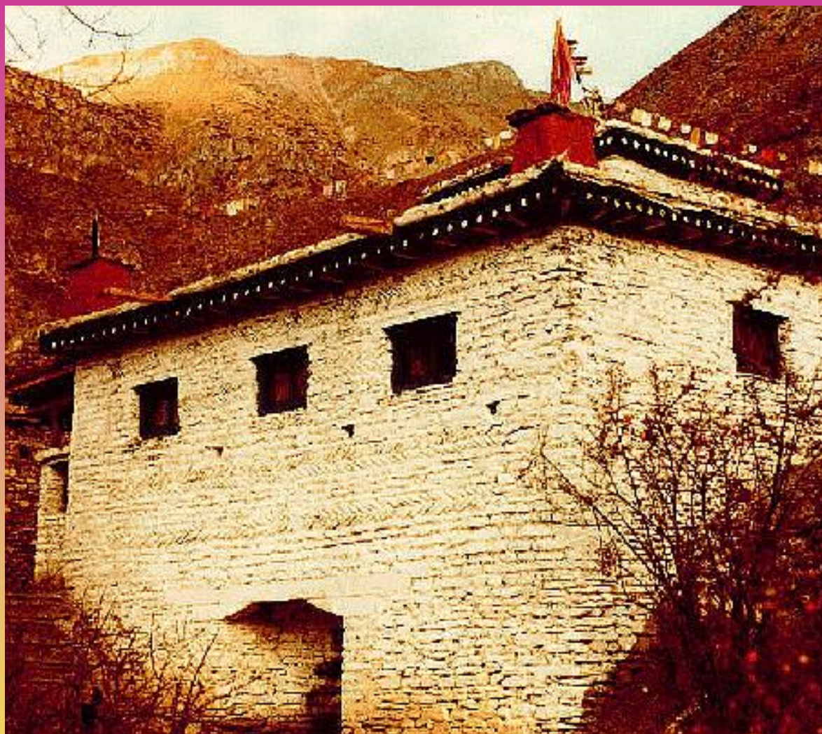
The “Temple Of Miraculous Fire” at Muktinath, Nepal. Photo by Ken Street.
